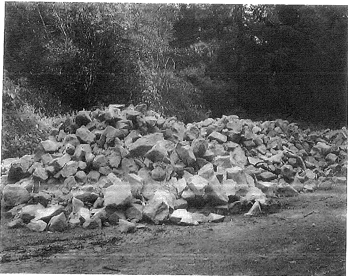
Stockpiled Malvern Stone ready for re-use
