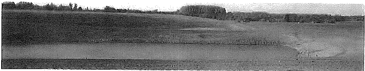
Landscaping as part of site restoration at Ball Mill Quarry, Grimley
