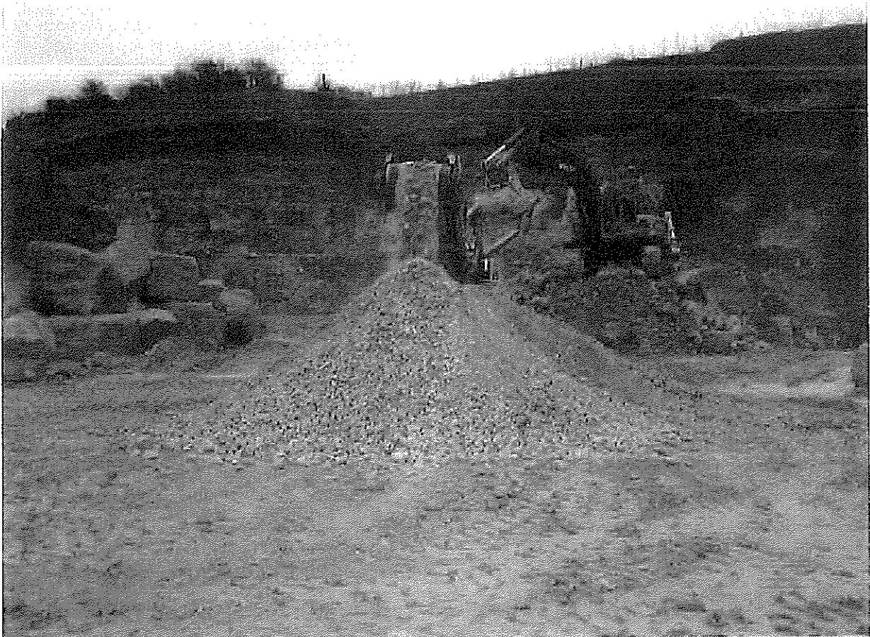
Processing crushed rock at Fish Hill Quarry
