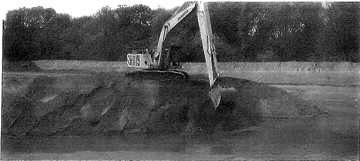
Working terrace sand and gravel deposits at Ball Mill Quarry (courtesy of Herefordshire and Worcestershire Earth Heritage Trust)
