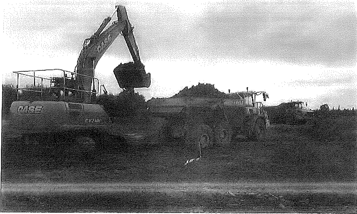
Excavating sand and gravel at Ryall's Court Farm Quarry
